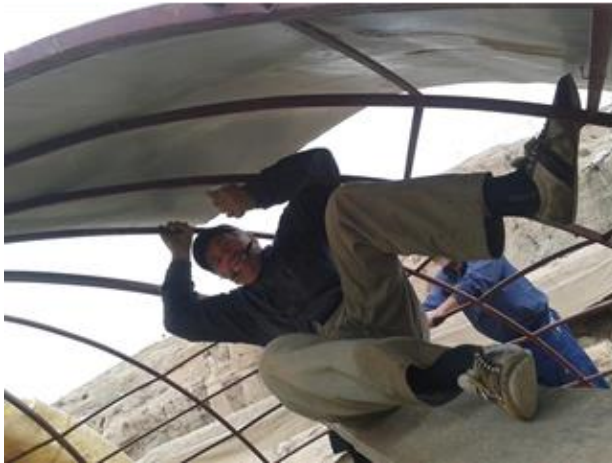
Fig. 2: First day of work on the abi dome
