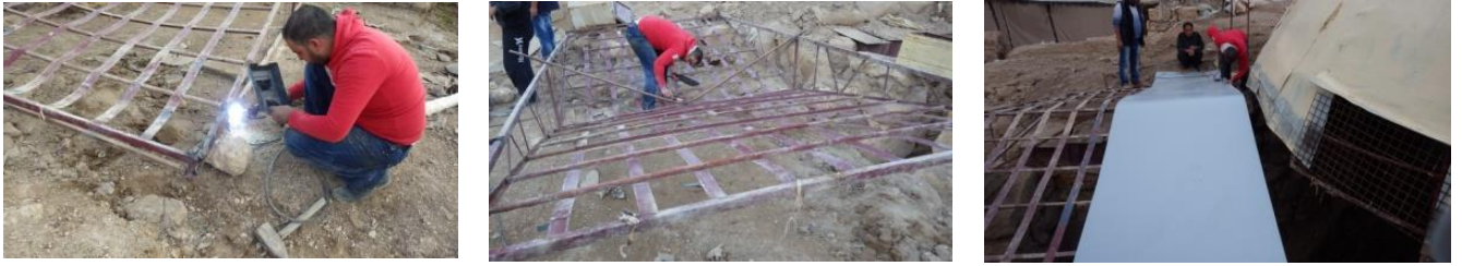
Fig 8: Different stages of work on the entrance
