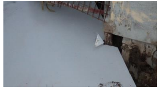
Fig. 9: Junction between metal sheets of the entrance covering and those of the abi dome
