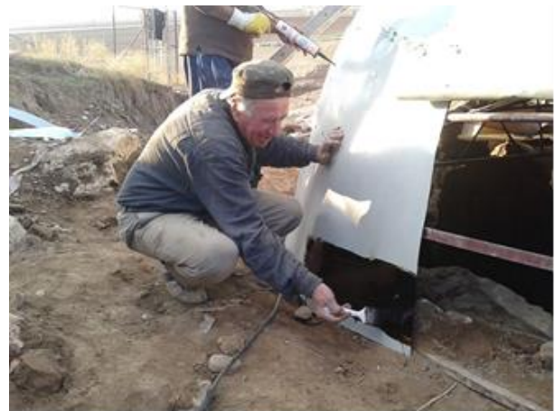
Fig. 3: applying pitch at the base of the Dome
