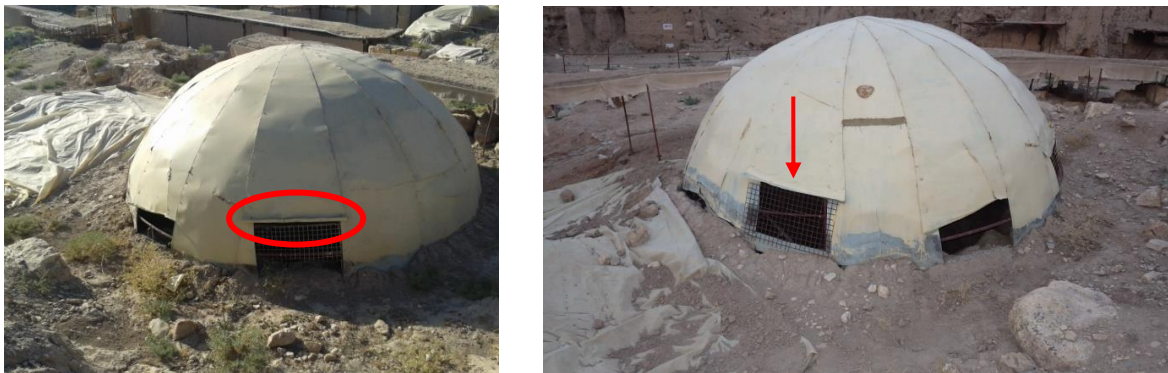
Fig. 5: Showing the openings and the drains above the openings
