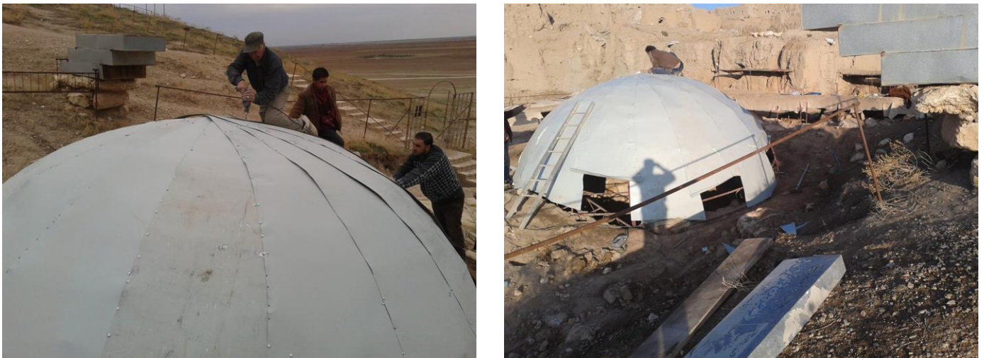
Fig. 4: Sabah Khasseem at work (left) and detail of the openings at the base of the new abi dome
