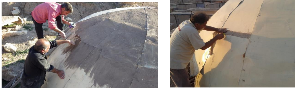
Fig. 6: Covering half the dome with dirt (6a, on the left) and the experiment with burlap (6b, on the right)
